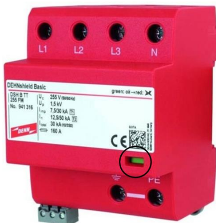
Figure 46: Check of overvoltage protection
