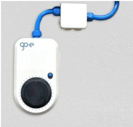
If necessary due to local conditions, lay additional supply line. When dimensioning the cross-section of the additional supply line, special attention must be paid to the method of installation. We recommend the following cable cross-sections, but the electrician has to decide according to the local situation:
